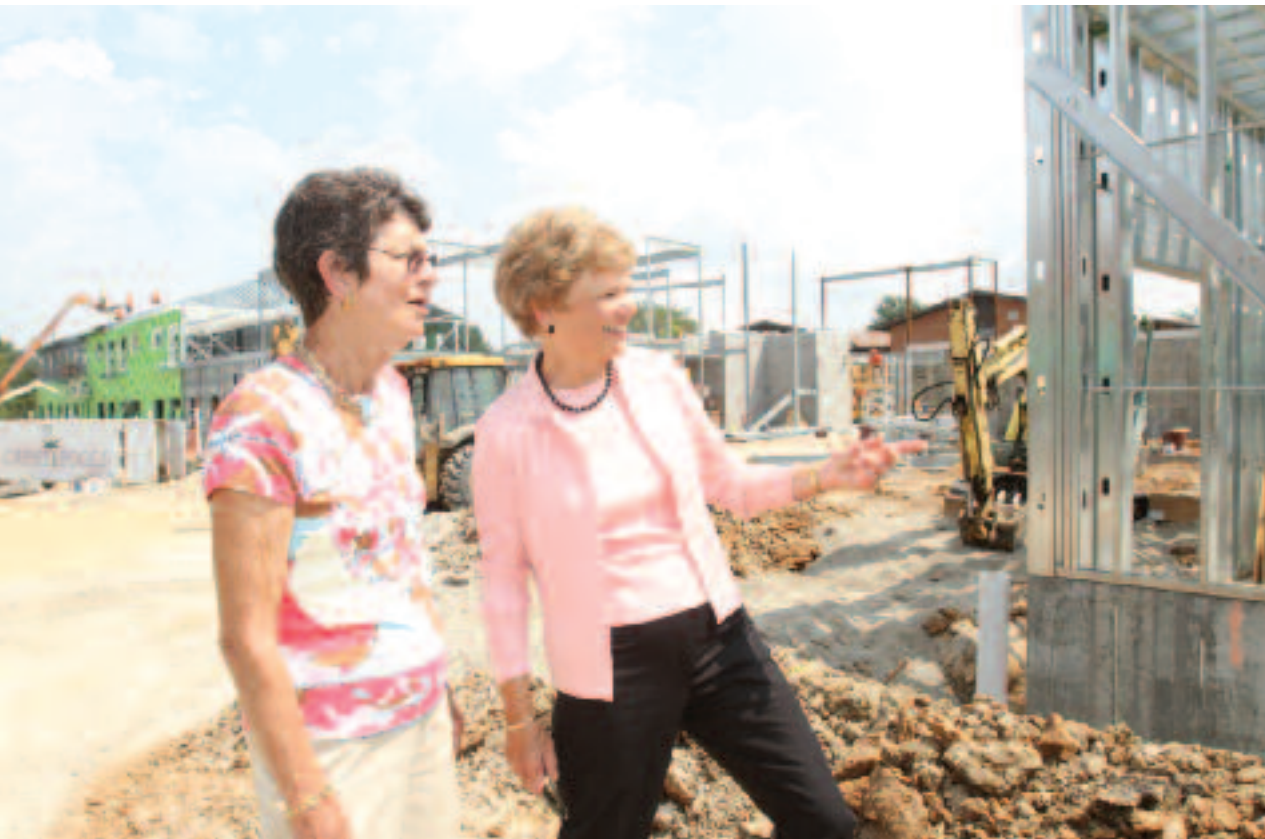
Sally Lilly and Marian Clifford tour the construction site of Charless Village.
